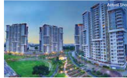
GREENAGE Hosur Main Road, Bengaluru
